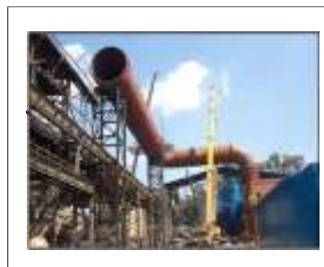
Installation of Large Bore Ducting
