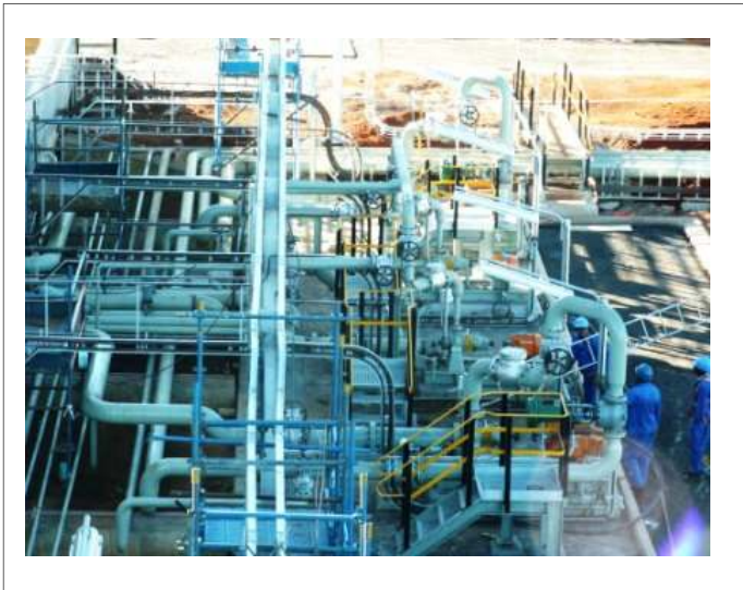
Petro-chemical pipework installation
