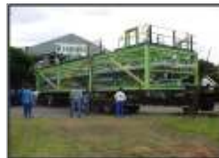
Metering Skid—Structural Steelwork and Piping by Arminco
